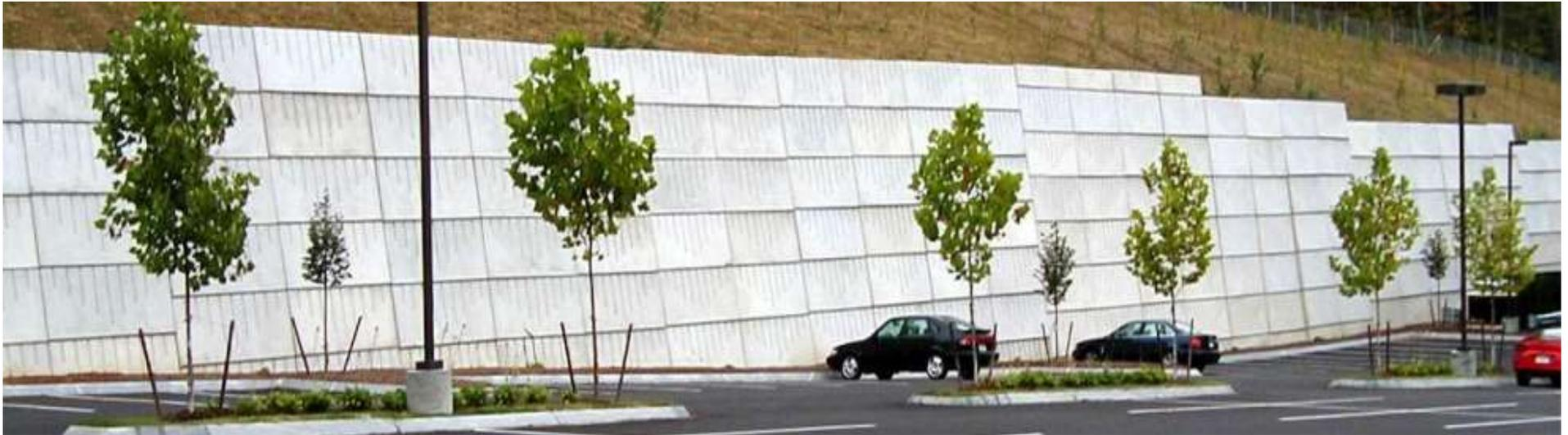
**Typical EVERWALL application: a gravity retaining wall to support a hillside and expand a needed parking area.**
