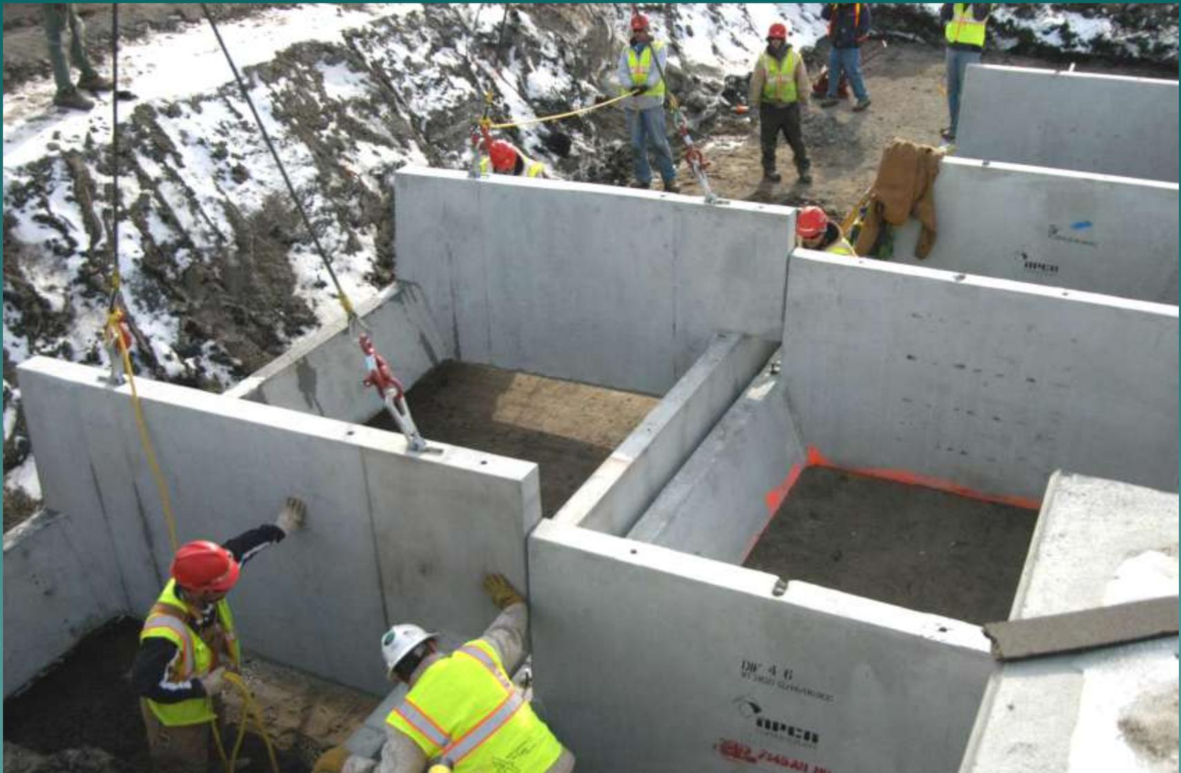
Slide back unit down along back of front unit
