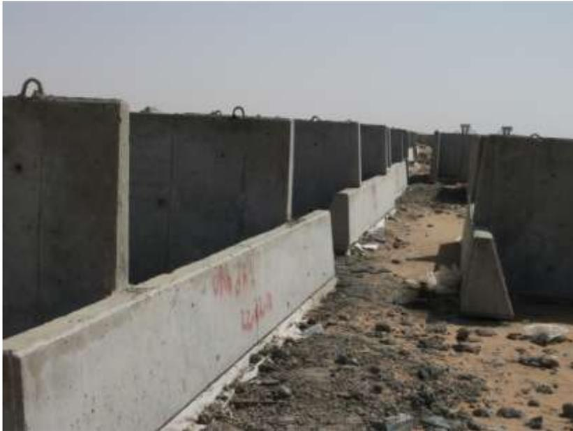
**Field Fabrication - of Units to Limit Transport to 100 miles**
